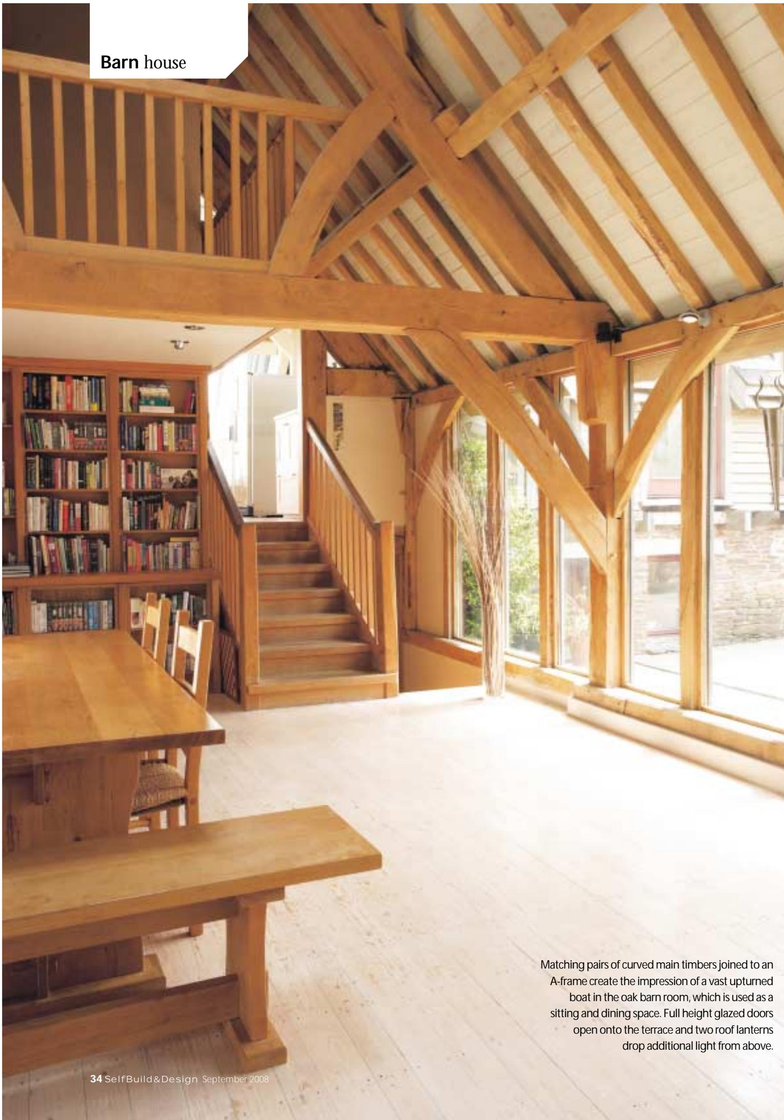
Matching pairs of curved main timbers joined to an A-frame create the impression of a vast upturned boat in the oak barn room, which is used as a sitting and dining space. Full height glazed doors open onto the terrace and two roof lanterns drop additional light from above.
