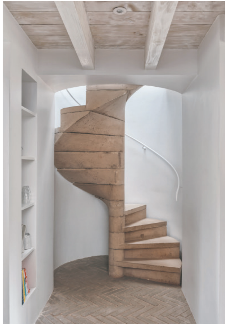
STAIRS Designed by Neil, and made by the builder from concrete using formwork, a unique spiral staircase winds up to the first floor.
