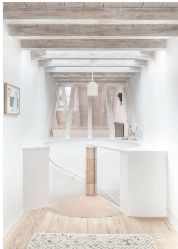
STAIRS Designed by Neil, and made by the builder from concrete using formwork, a unique spiral staircase winds up to the first floor.
