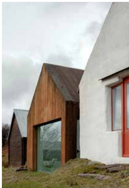
LEFT The modern extension, designed by Urban Agency, added to the rear of the original cottage and linked by a glazed walkway, is in fact made of poured concrete. RIGHT The cottage overlooks Carragh lake, near Glenbeigh in Kerry.
