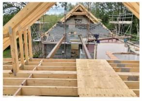
ROOF AND SUBFLOOR With the walls in place, the subfloor and roof framework were constructed.
