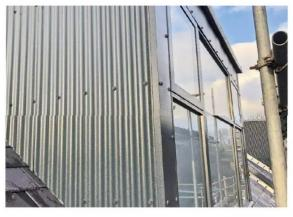
STEEL DORMER The dormer was clad in corrugated steel in dark grey to match the aluminium frames.
