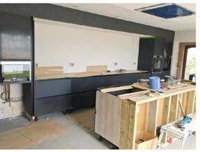
KITCHIEN INSTALLATION Once the concrete floors had been laid, the kitchen units, from Howdens, could be installed.
