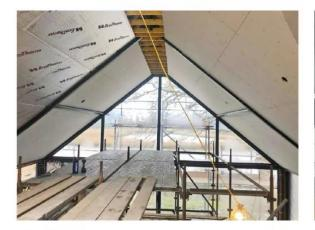
INSULATION SCAFFOLDING Internal scaffolding was required for the insulation and plasterboarding of the extension.
